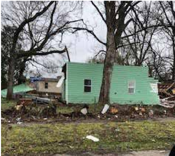
Tornado damage near the Bosco Nutrition Center in Selma, AL
